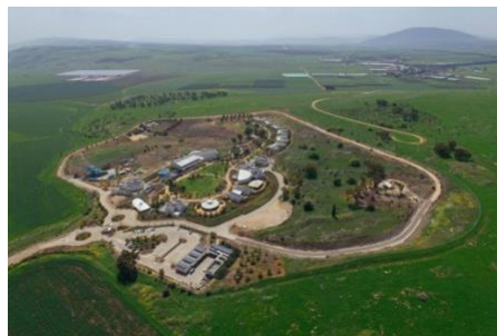
Jordan River Village Campus (photo courtesy of Jordan River Village)
